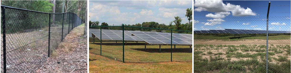
Above: Chain wire mesh; black coated (left), green coated (centre) and uncoated galvanized (right)
