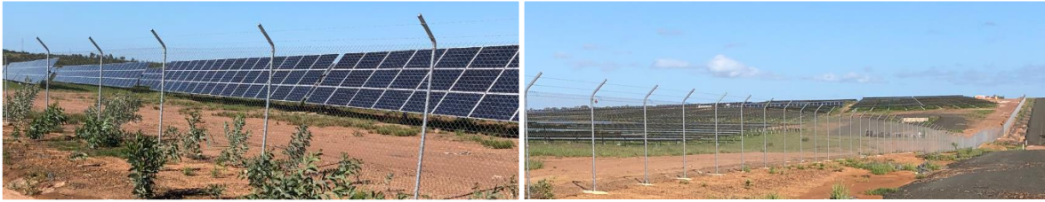
Above: Solar farm boundary fences installed at FRV solar farms in Australia (taken during construction)
