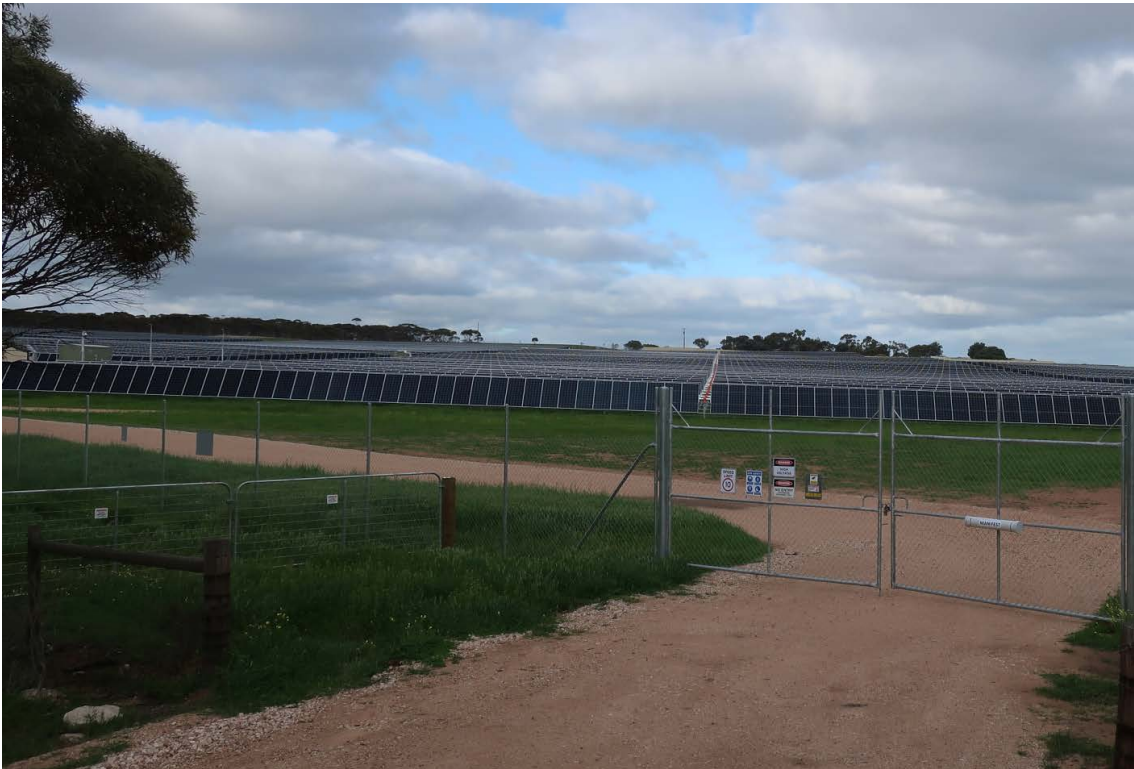
Plate 1: Perimeter fencing at Terregra Solar Farm at Murray Bridge
