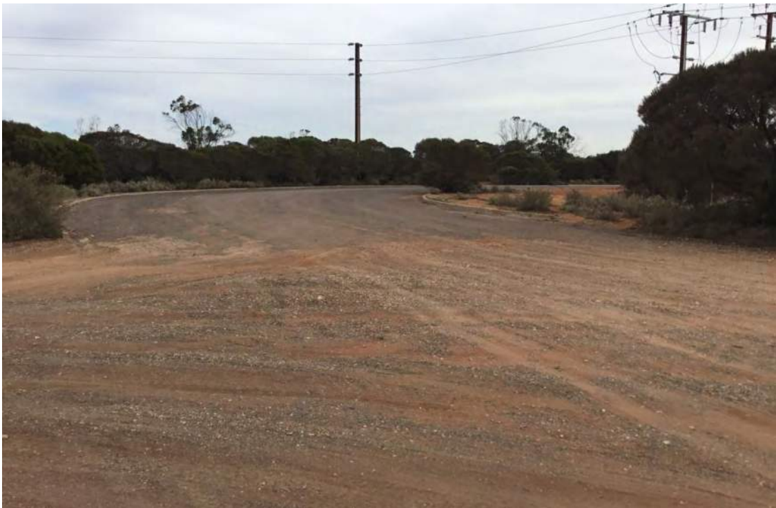
Figure 4-6 - Existing pavement condition adjacent proposed access point
