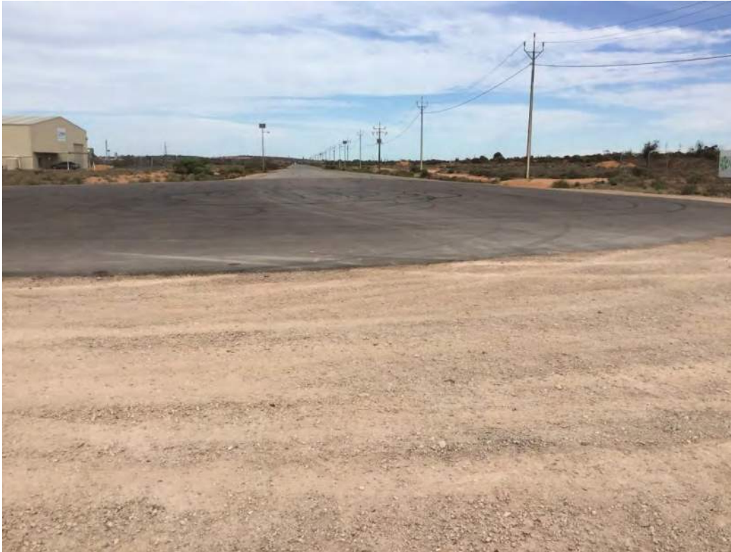
Figure 4-16 - Current condition of Cul-de-sac
