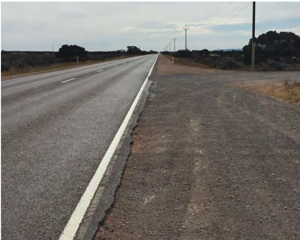
Figure 4-13 – Existing condition of pavement at Lincoln Highway Access Point
