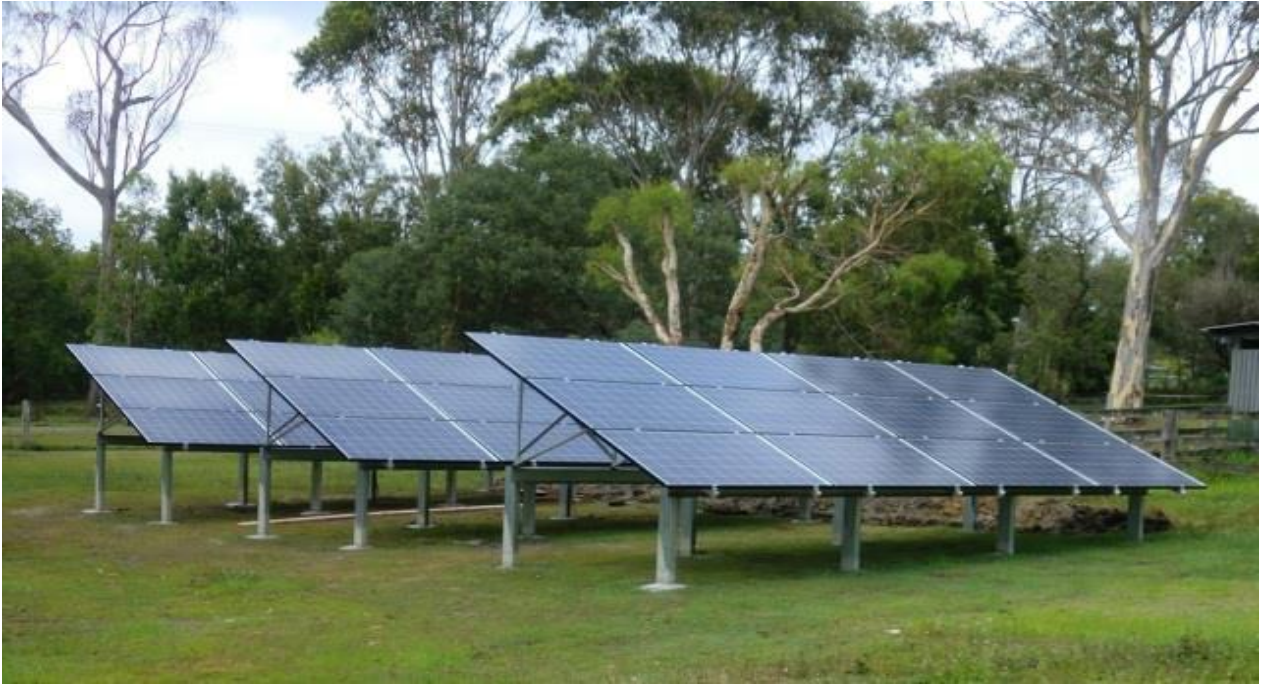
Figure 9. Typical Ground-mounted Solar Panel Layout
