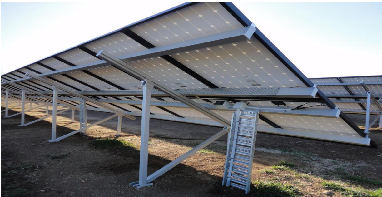
Figure 8. Typical Ground-mounted Solar Panel Layout
