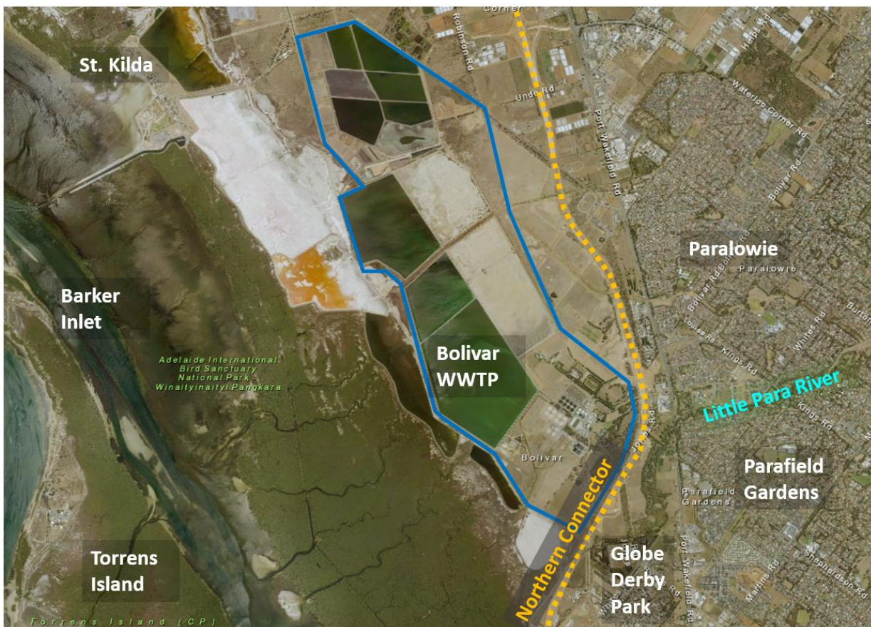
Figure 1. Bolivar WWTP and surrounding land uses. Base image source: Location SA Map Viewer, http://location.sa.gov.au/viewer/#
