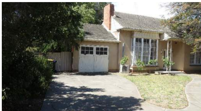
Front yard, 38 Glenrowan Road
