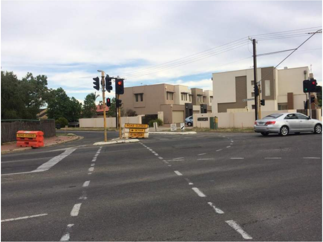
Figure 8: Glen Rowan Road closed due to road works
