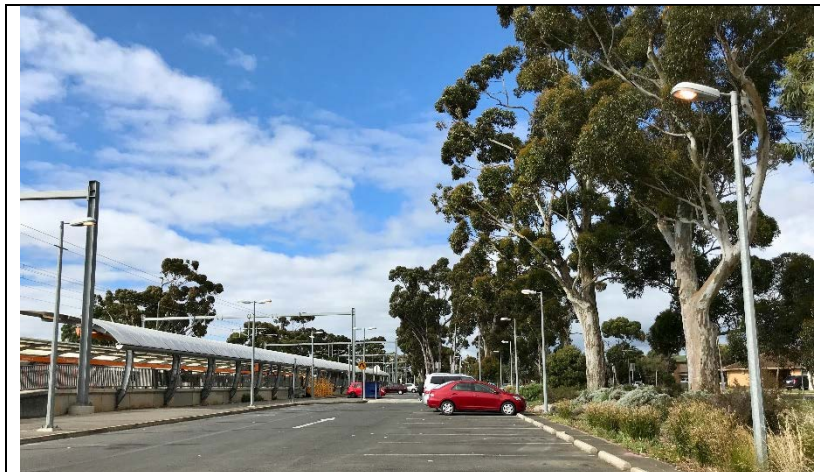
Figure 11: Looking North West of Station and Car Park off Crozier Terrace
