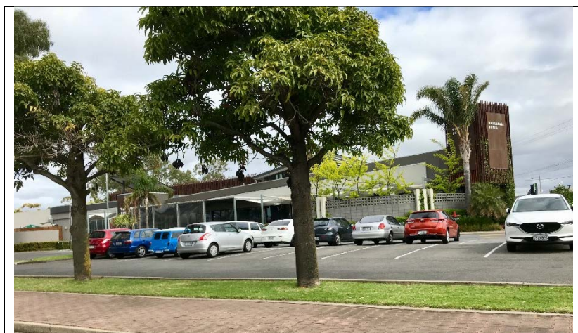
Figure 21: Warradale Hotel looking South from Prunus Street
