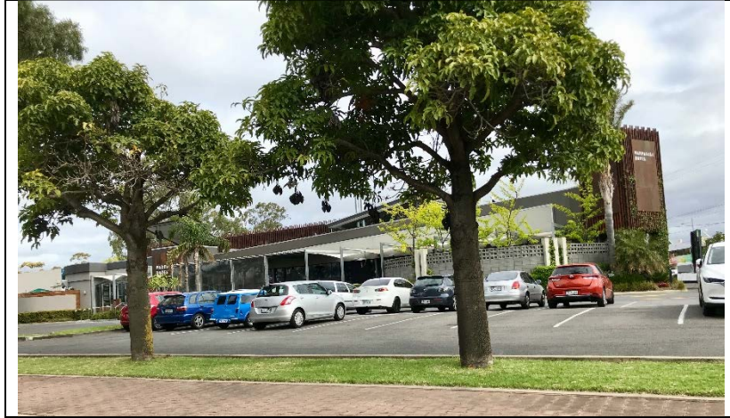
Figure 22: Warradale Hotel looking South from Prunus Street
