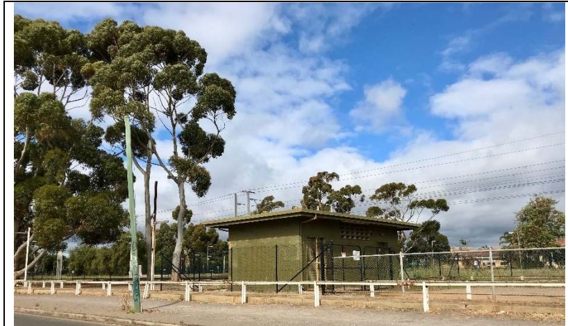
Figure 16: Existing Railway Building North East of Station from Murry Terrace
