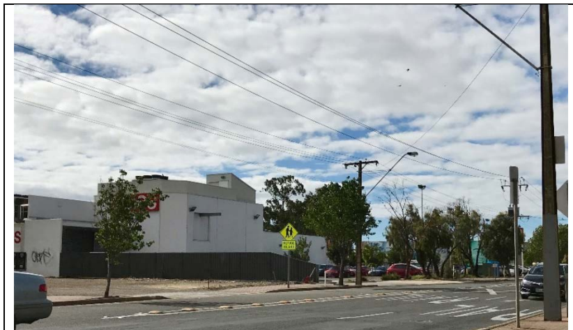
Figure 20: Rear of Coles Supermarket from Morphet Road/Murray Terrace Intersection
