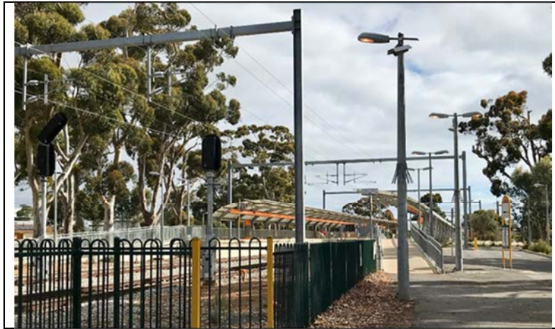
Figure 2: North West end of Oaklands Station from Pedestrian Crossing
