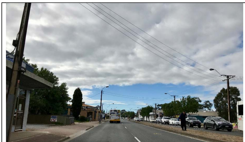
Figure 24: Oaklands Road looking North East from Railway Terrace
