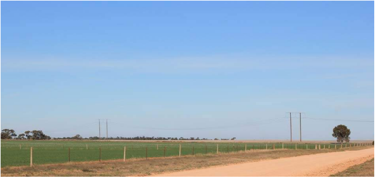
Figure 7: View of the existing transmission line running through the proposed development site
