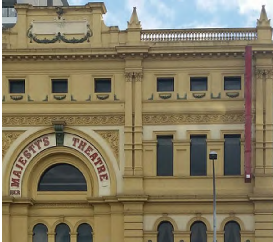
02 EXISTING GROTE STREET HERITAGE FACADE
