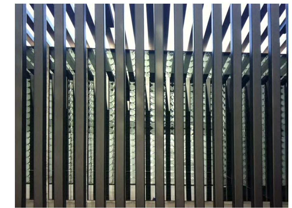
EF03 BLACK POWDERCOATED ALUMINIUM FINNS TO FACADE OR SIMILAR.
