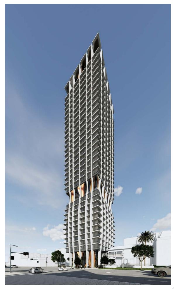
The architectural language of the tower inverts the typical structure of a modern tower. It takes the typically clad building in lightweight panels of glass and metal, and draws the structure to the facade line.
