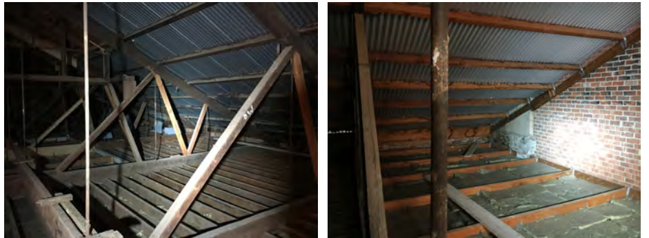
IMAGES 06 & 07 – Photos taken within roof space showing altered trusses, 'new' purlins and 'new' ceiling joists (C&G).
