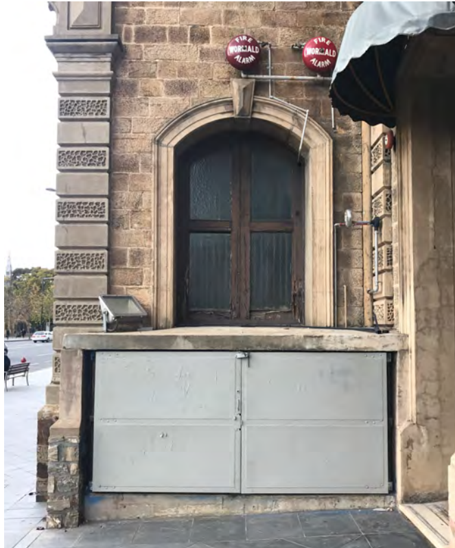
IMAGE 11 – Fire Booster Box.
