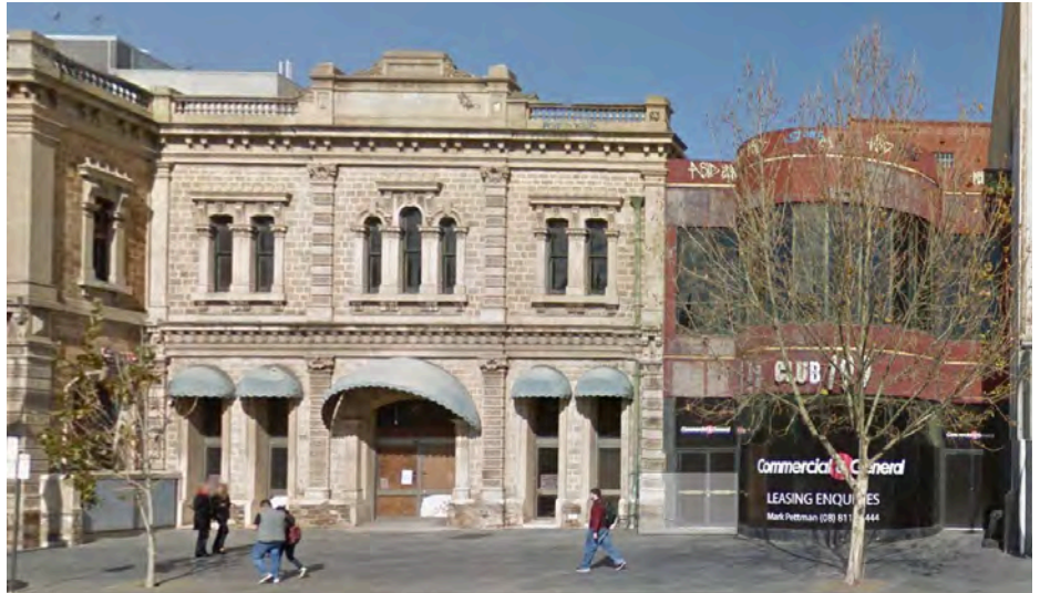
IMAGE 10 – North Facade showing Fire booster box, canopies and lower levels windows and doors.
