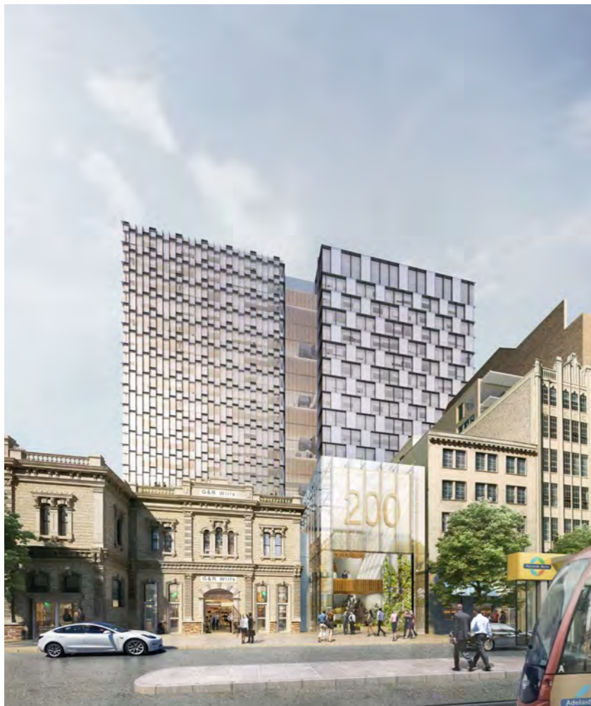
NORTH TERRACE ENTRY
