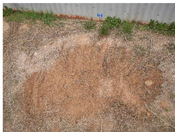
After - Subsequently the area was raked and checked for other possible fragments – no asbestos was visible
