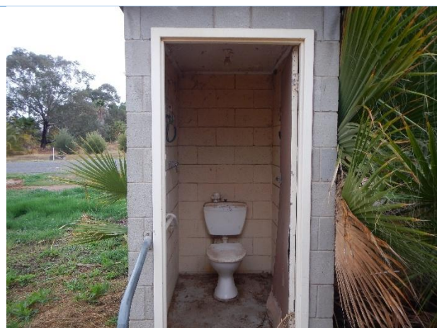
Example: External/Internal paint to Residence Outhouse
