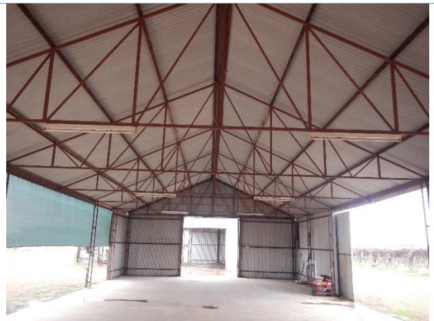
Example: Internal paint to structural steel frame of Shed 3
