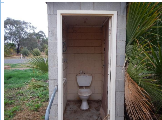
Example: External/Internal paint to Residence Outhouse
