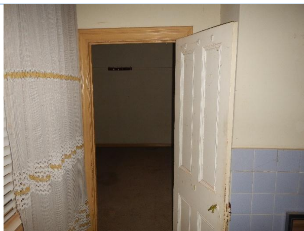
Example: Internal paint to Residence
