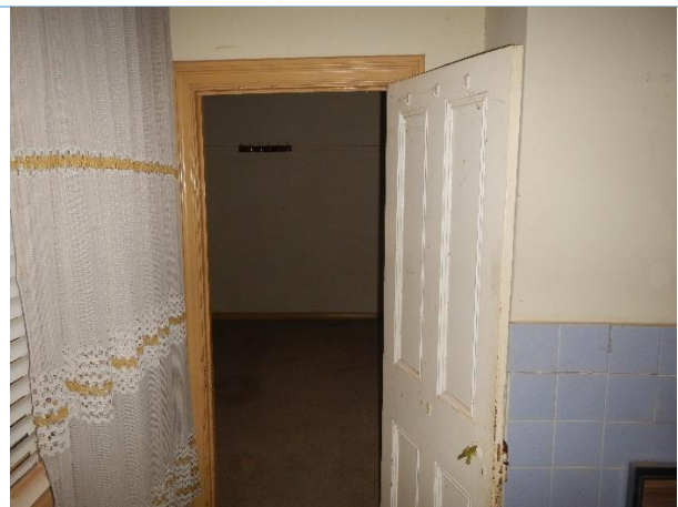
Example: Internal paint to Residence
