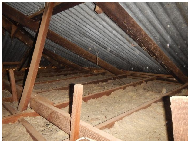
Example: Ceiling insulation over ceilings to main roof of Residence
