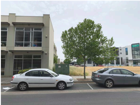
VIEW OF EXISTING TRANSFORMER
