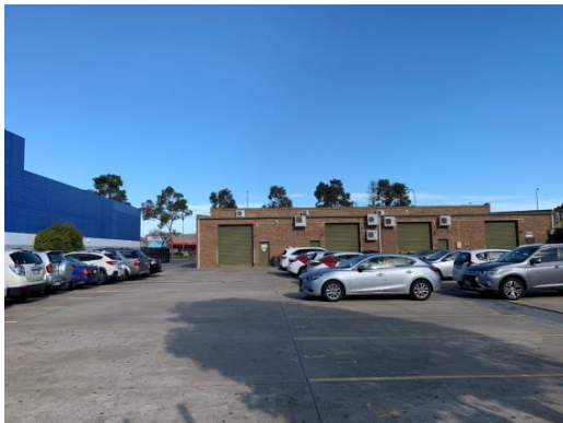
Within the rear car park, looking south with the driveway access on left
