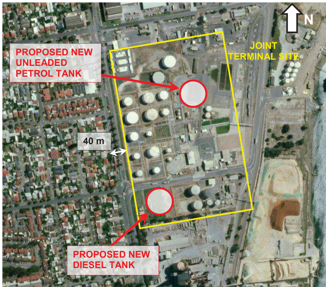
Figure 1-1: Aerial image showing location of Joint Terminal site with surroundings (source: ArcGIS Earth).
