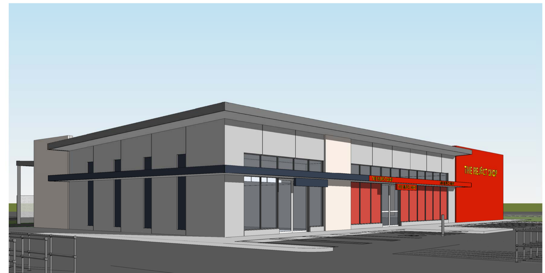
View from West
