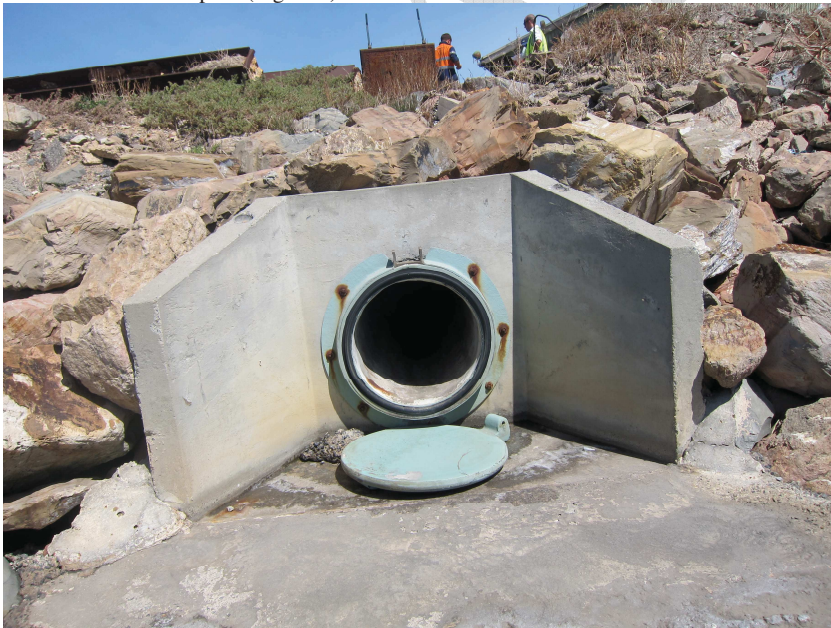
Photo 3 – northern outfall for the surface run off from the catchment area on the western side of the sheds and Port River (Figure 2).
