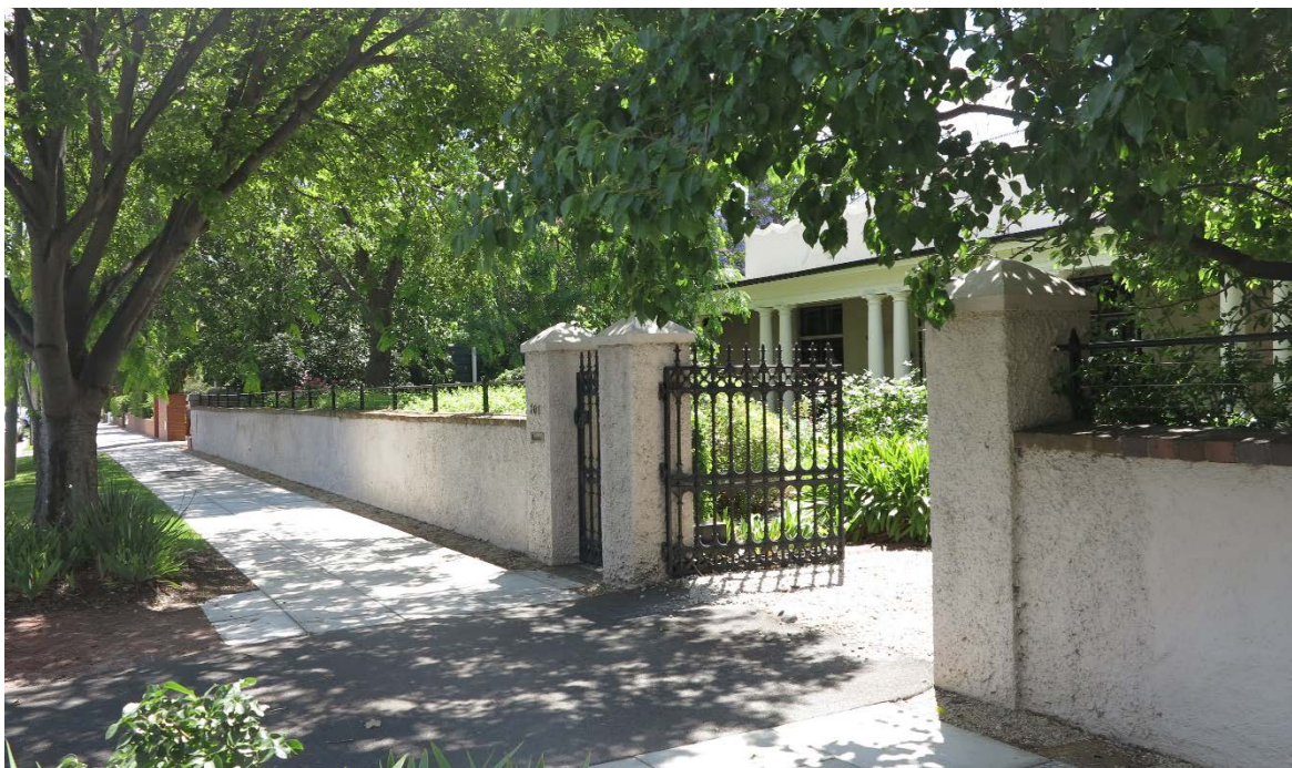
View of the existing dwelling at 306 Ward Street.
