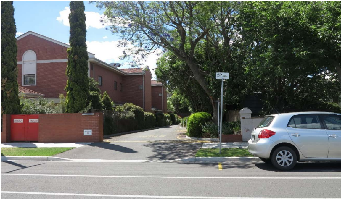
View of the eastern wing of Calvary North Adelaide Hospital (Mary Potter Hospice) and existing driveway which adjoins 306 Ward Street.
