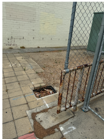
FIGURE 4: EXISTING TELSTRA PIT
