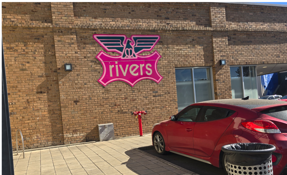
Figure 15: Onsite Fire Hydrant
