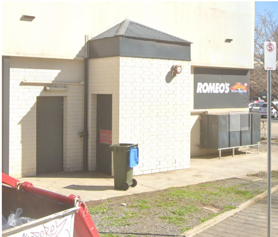
Figure 16: Sprinkler Valve Room
