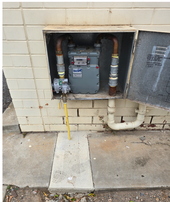
Figure 7: Gas Meter
