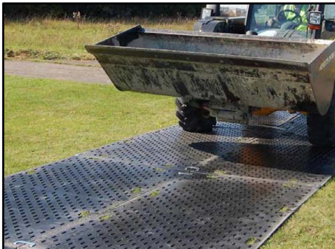
Left: Track mat ground compaction mitigation (image https://www.rampchamp.com.au/ )
