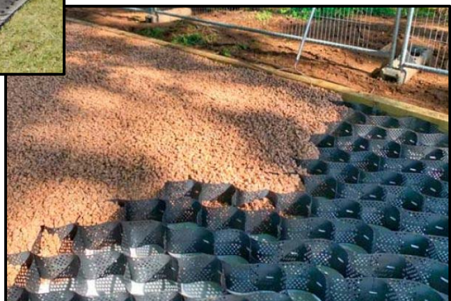
Right: Geoweb ground compaction mitigation (image www.greenfix.co.uk )
