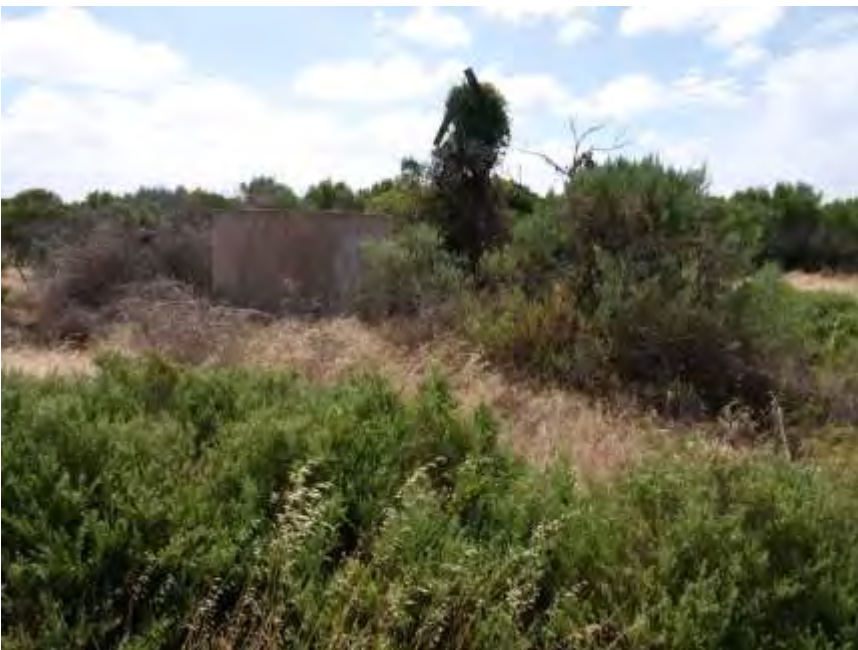
Photo 3 Water tank and windmill (near E706446 6107219) north of proposed glamping tent location
