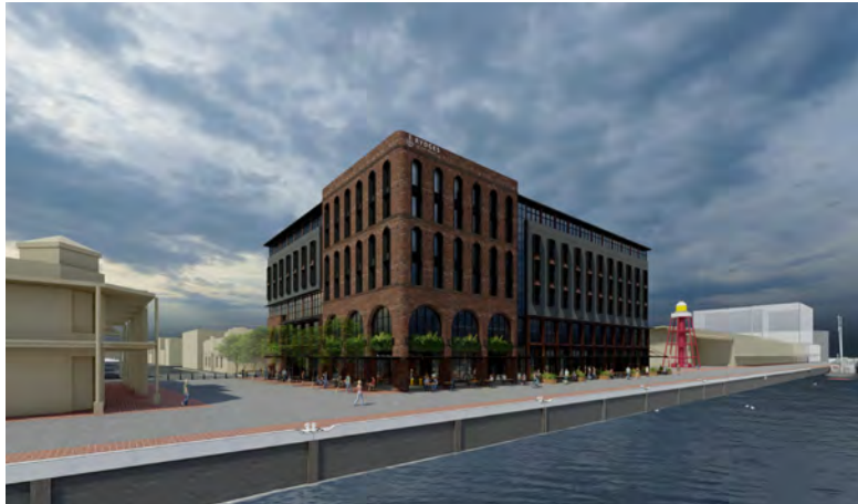
McLaren wharf looking south-west
