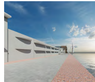
McLaren Wharf near Warrawee Dock
