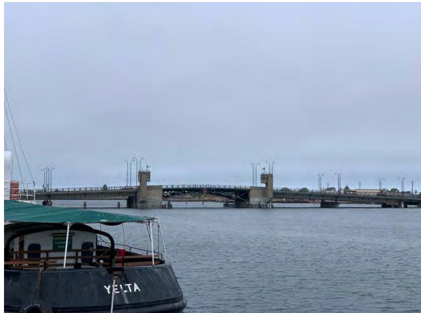
IMAGE 12 – Photo of Birkenhead Bridge from near the Subject Site (Bridge is a State Heritage Item) (by Author).
