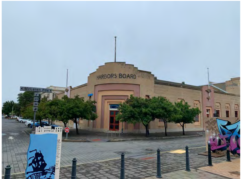
IMAGE 07 – Photo of building directly opposite site on McLaren Parade (within State Heritage Area) (by Author).
