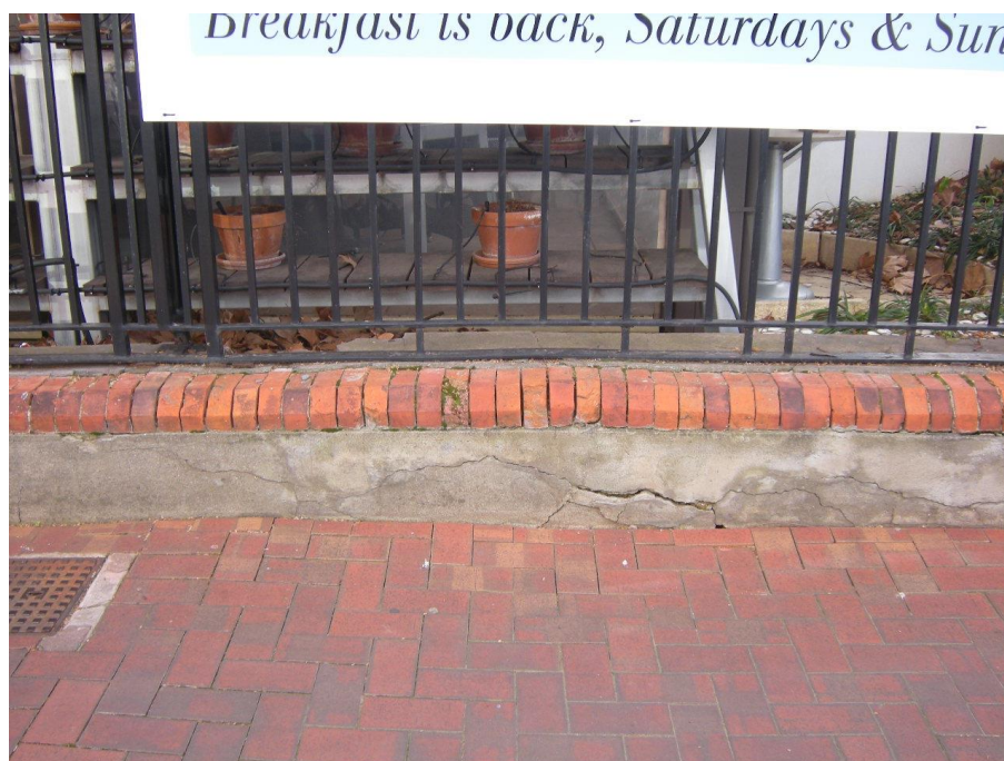
O'Connell Street frontage – displaced fence base
