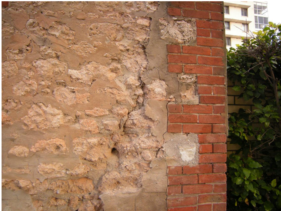
Stables - northern wall displacement on Ward Street
