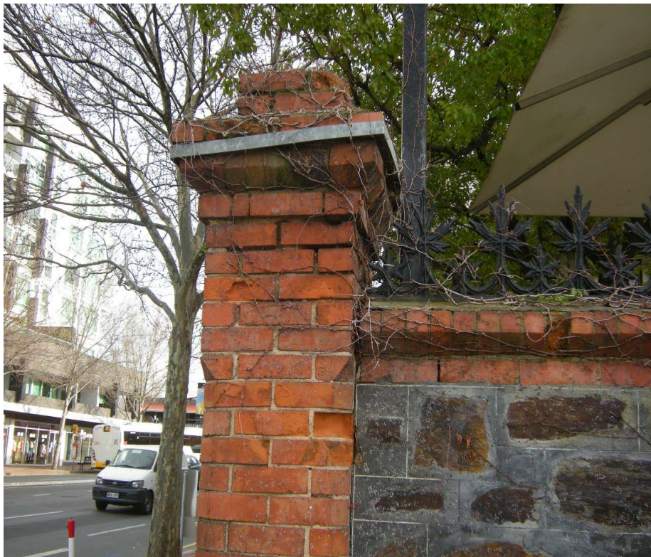
O'Connell Street corner – dilapidated fence pillar
