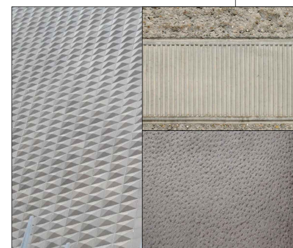
LIGHT COLOURED PRECAST CONCRETE - TEXTURED
