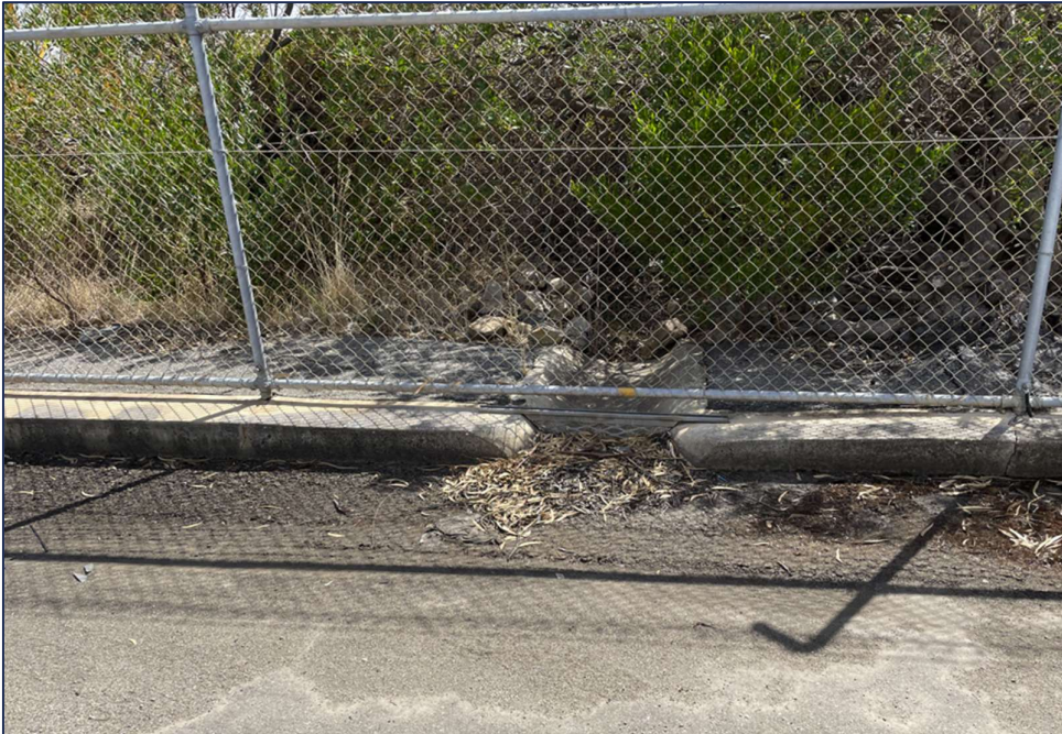
Figure 6 Site Inspection Photo: Sub-station existing kerb outlet
