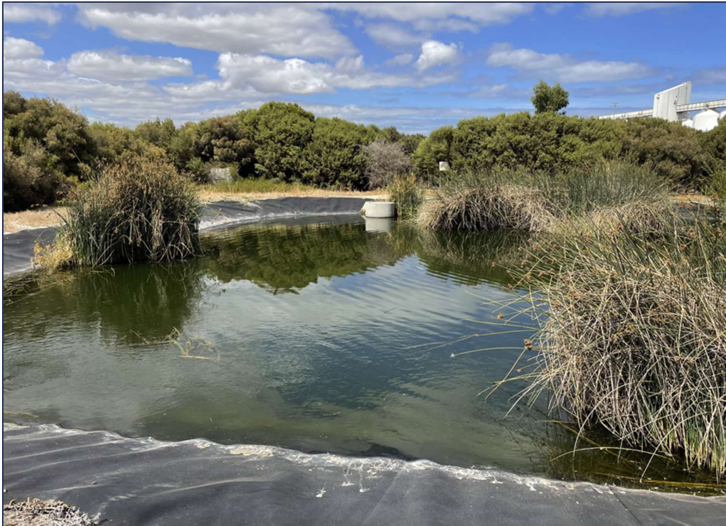
Figure 7 Site Inspection Photo: Existing Stormwater Basin
